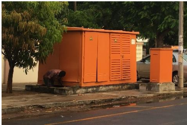
Figure 7.4-2 Transformer for underground line (315kVA)
