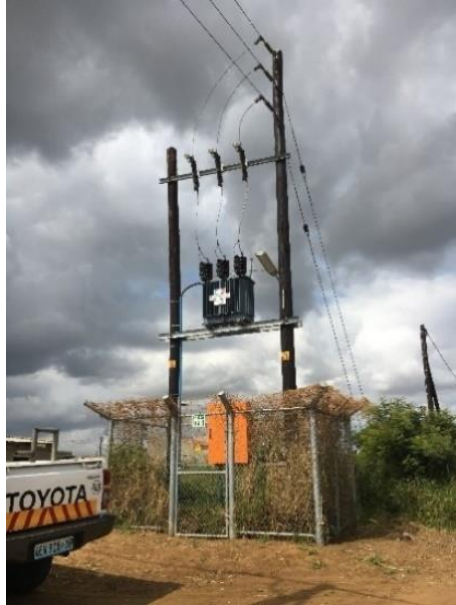
Figure 7.4-1 Transformer for overhead line (100kVA)
