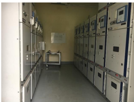
Figure 7.1-5 Inside of PS (Left: Remote operation type, Right: Manual operation type)
